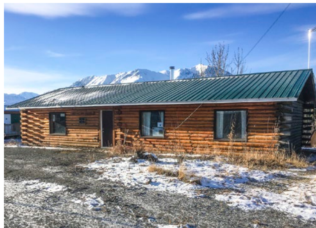
Walter Wood building, October 2017. Photo by M. Schmidt.
